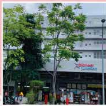
No.3, Soon Lee Street, #04-14, 16,17, Pioneer Junction, Singapore 627606
